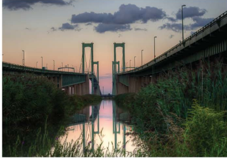
DELAWARE MEMORIAL BRIDGE August 1951
