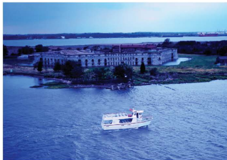
FORTS FERRY CROSSING March 1997
